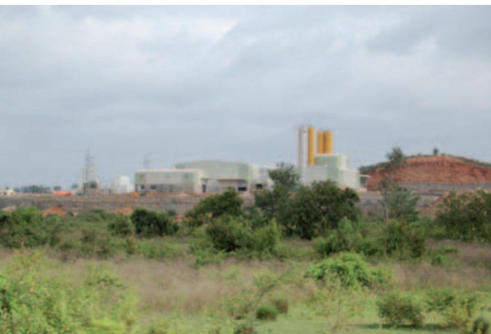
Building ground for Basant Betons
